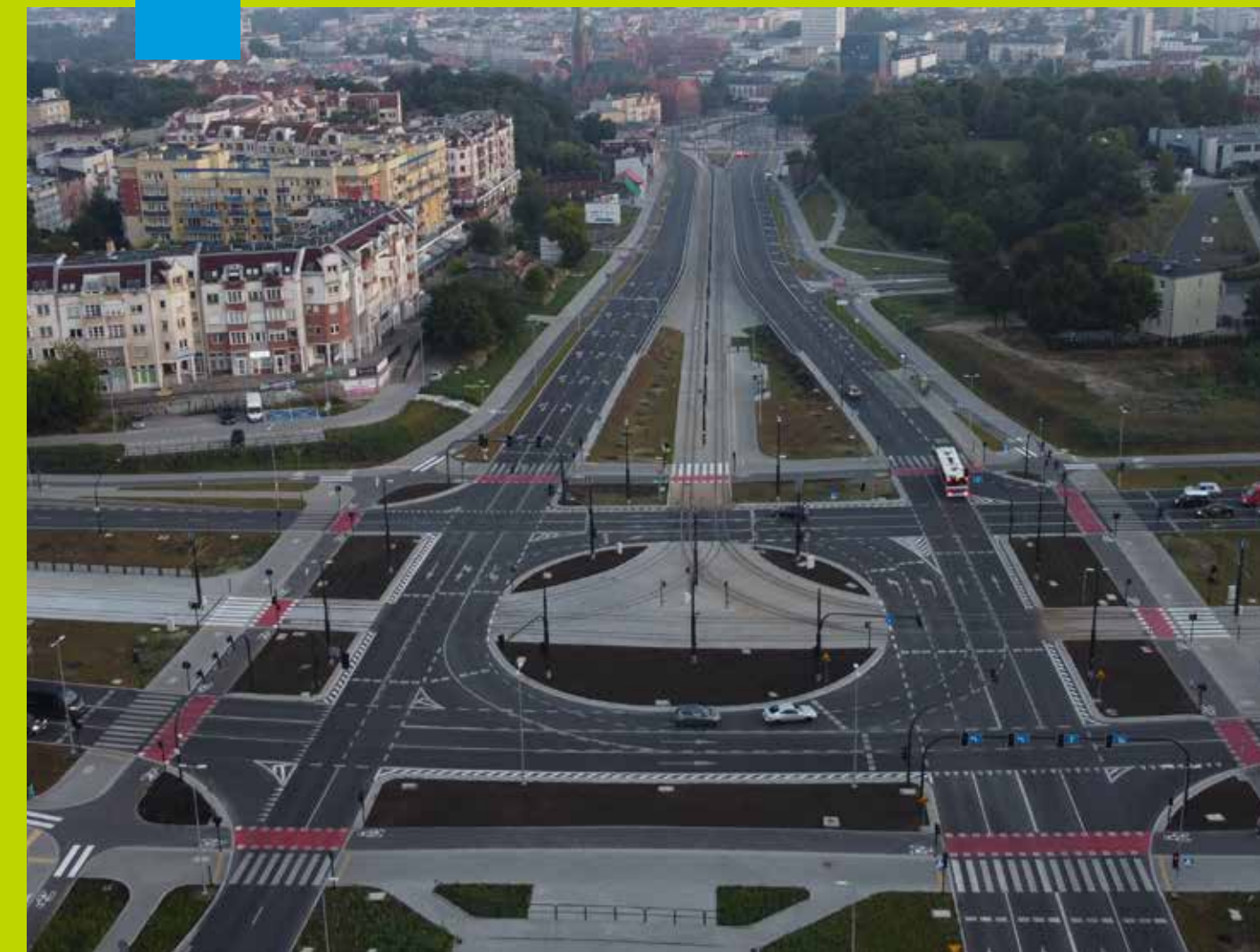
Construction of nearly 2 km of tram tracks. An increase in availability of public transport, reduction in noise contamination, construction of "Park&Ride" car parks and of over 4.5 km of cycling tracks with city bike stations, elements preventing access of small animals. Innovative use of solar energy to power active road signs with solar energy.
